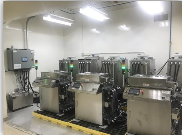
**Completely closed, modular system incorporating integrated heated storage containment tanks with a self-contained, automatic ultrasonic washer**
